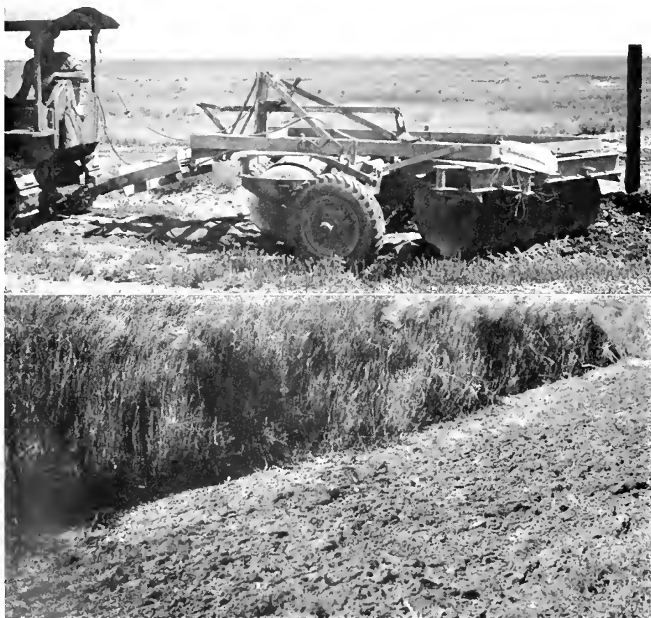
Disking roadside areas beyond ditch line establishes firebreaks
